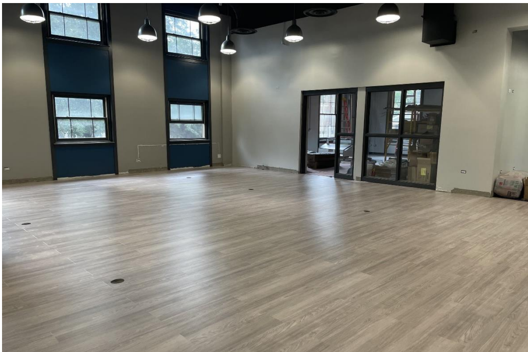
As you enter the main floor, you will notice the new flooring in the main makerspace area. The luxury vinyl flooring has a modern, clean look while providing a durable and easy to clean surface. Our office and closet spaces have also been tiled. With those spaces completed the vast majority of main level flooring is complete.
