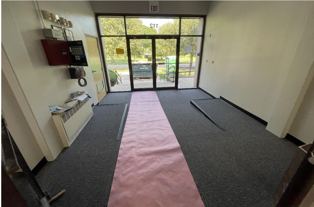
The reconfigured vestibule looks ready to welcome customers with the ADA ramp and new weather resistant carpeting.
