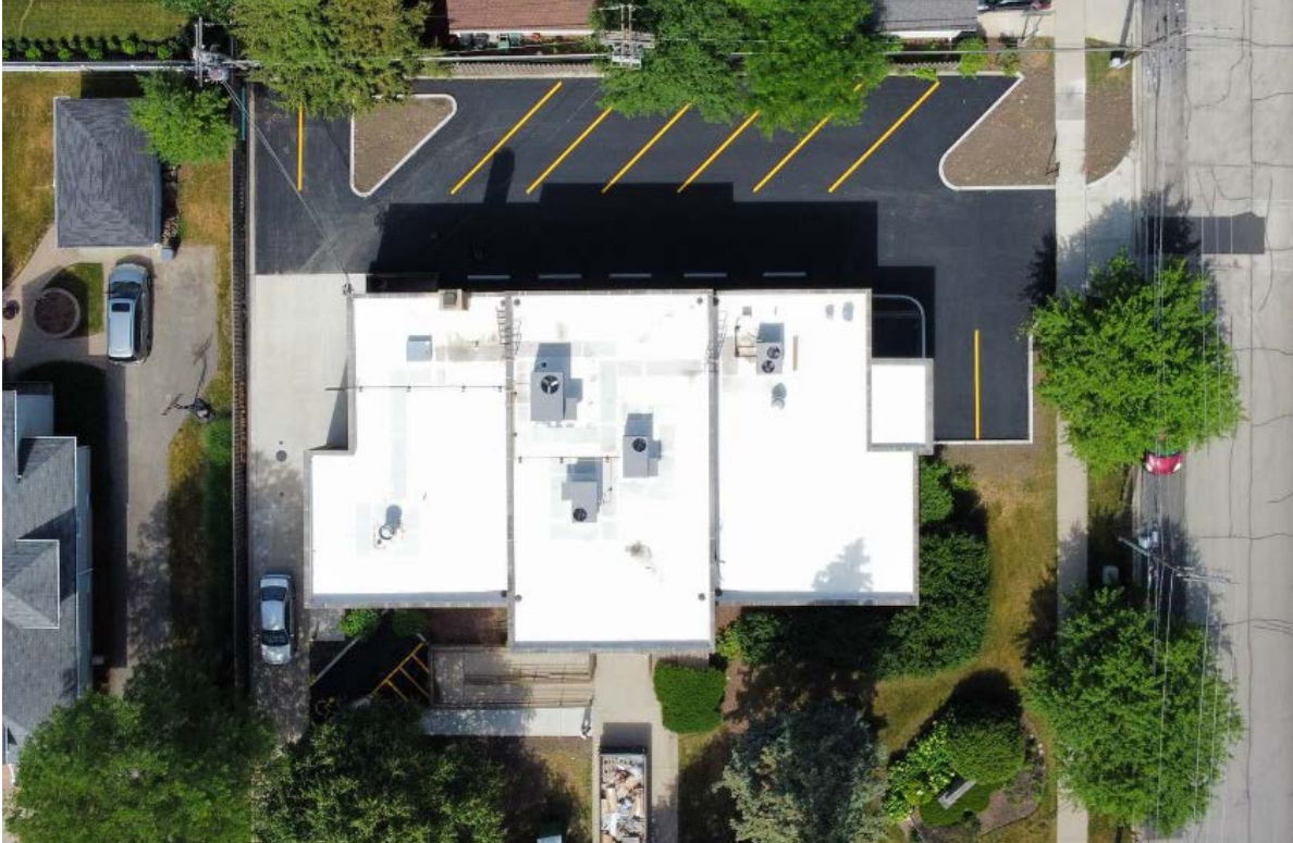
Aerial view of the striped parking lot. The reconfiguration of the lot increased the number of parking spaces from 7 to 12.
