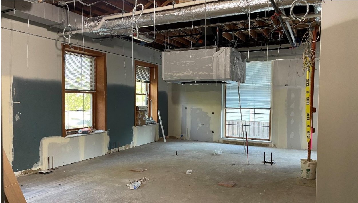
Kitchen walls are prepped and ready for the commercial kitchen paneling.
