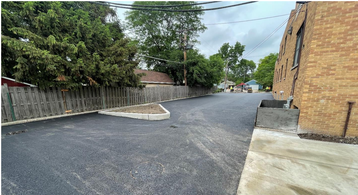
Reconfigured and repaved parking lot.
