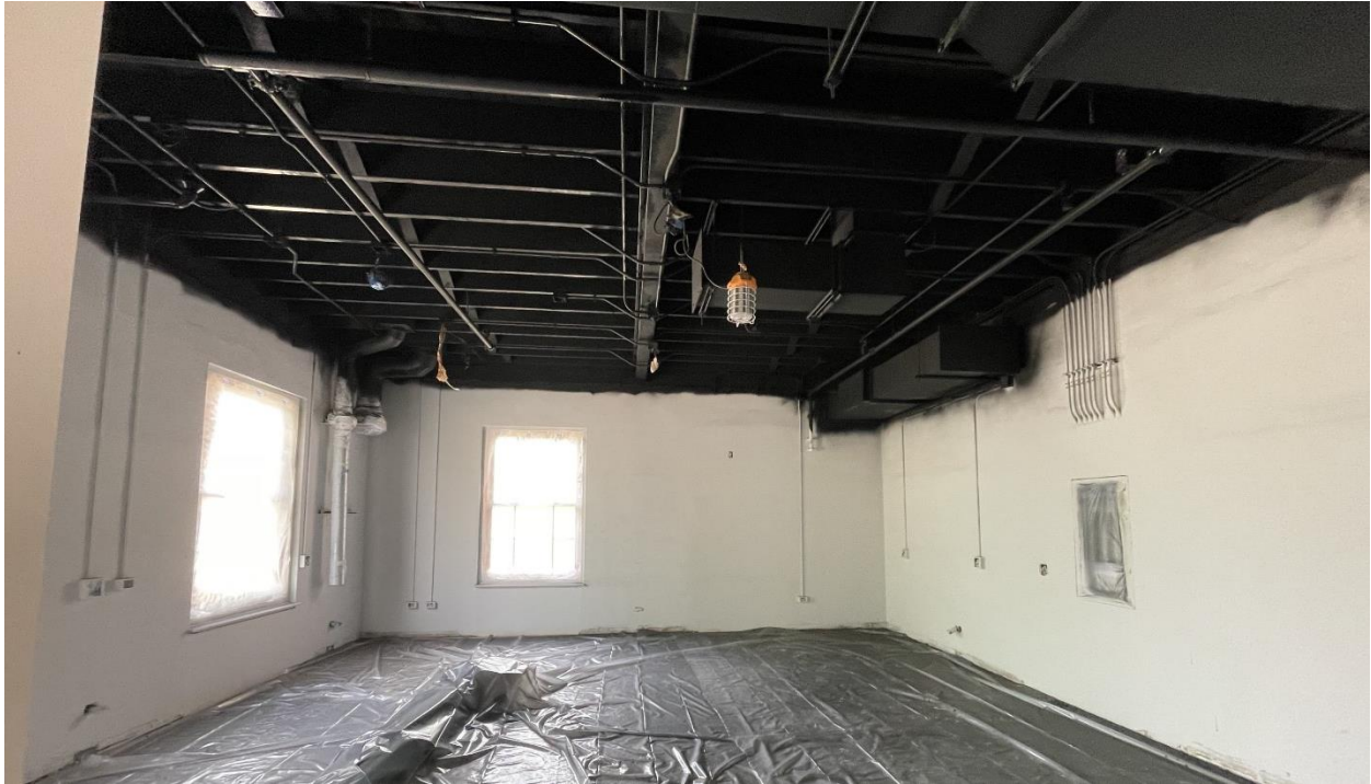
Painted ceiling and primed walls in the fabrication room.
