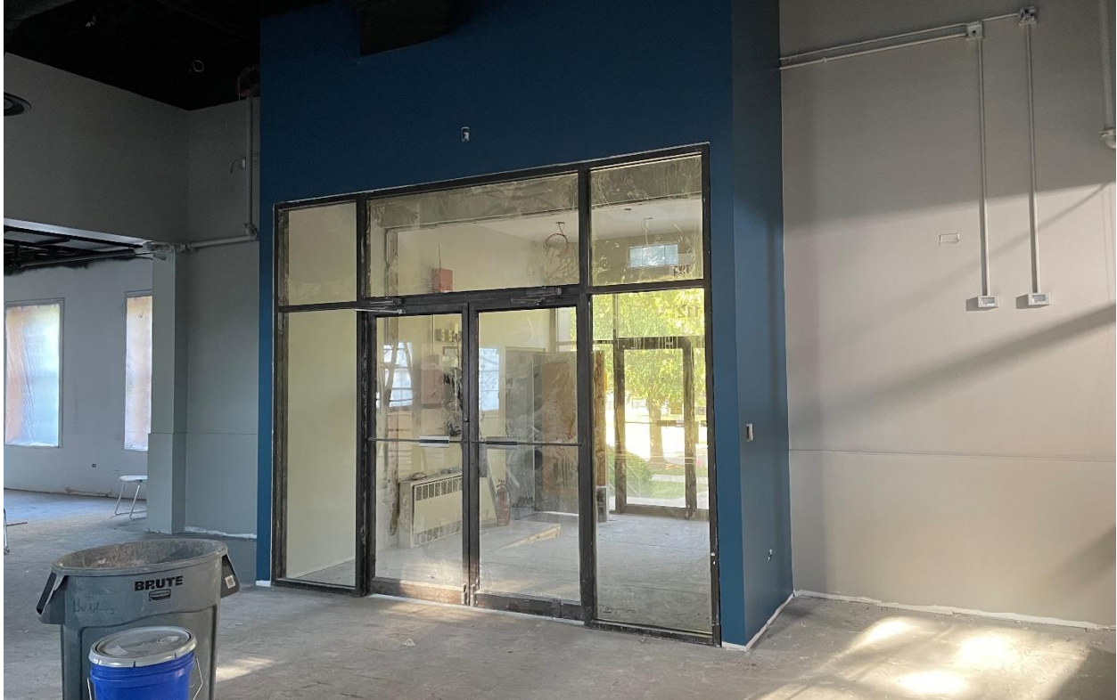
The vestibule reconfiguration included moving the doors into the space approximately 3 ft. The original doors and glass have been reinstalled in the new structure.
