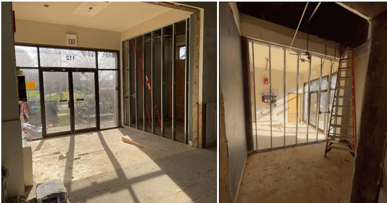
The new vestibule configuration allows for the ADA accessible ramp and storage space for the kitchen.
