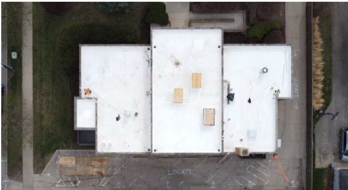
Aerial view of new roof
