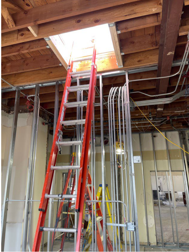
New roof hatch allows easier and safer access to the roof. Substantial electrical infrastructure has been completed and is currently in inspection phase.
