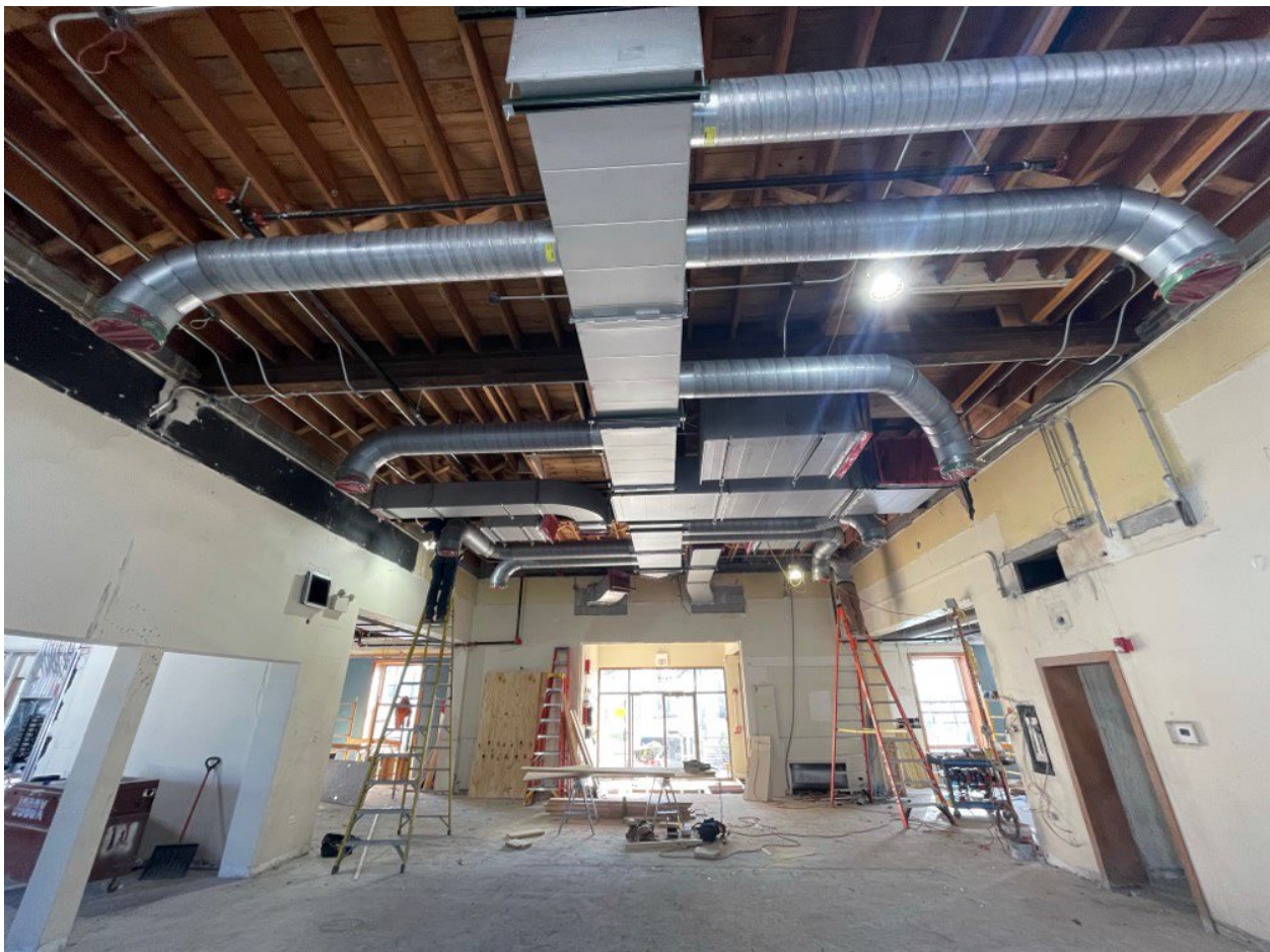
HVAC ducting has been installed throughout the building.
