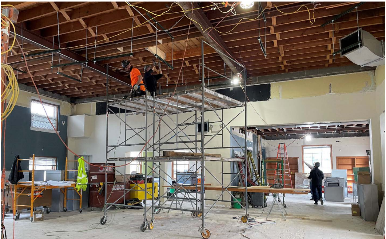
Main Makerspace area (Flex 1) and Flex 2 – electrical and HVAC installation
