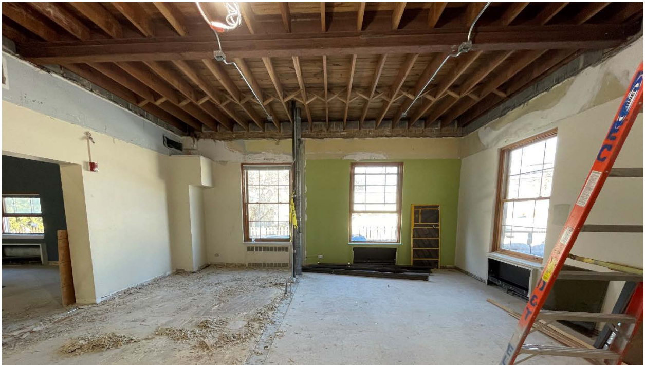
Industrial tools/equipment room
